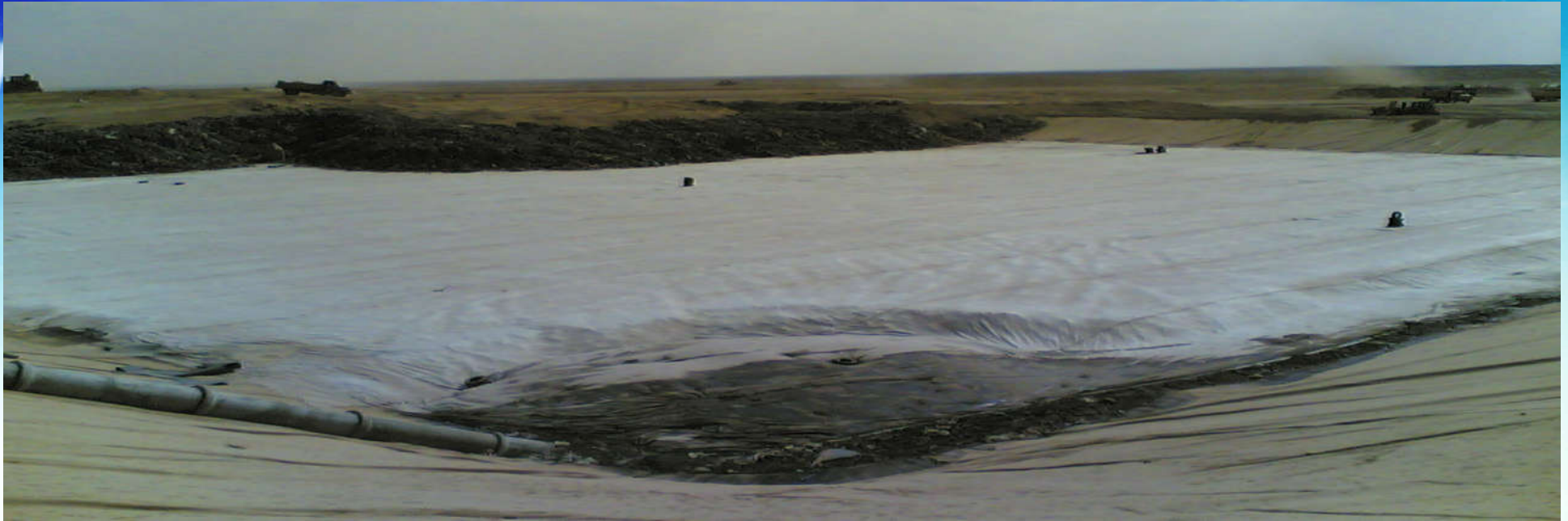
A layer of Geo-textile (180gm density) on top of pebble layer
