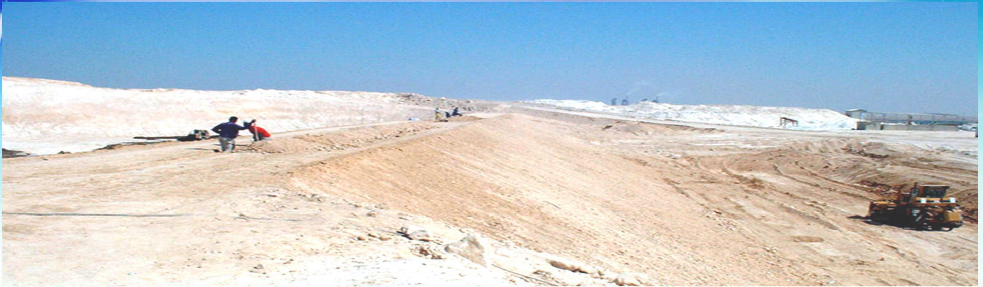
Excavation works and preparing cells to receive waste.
